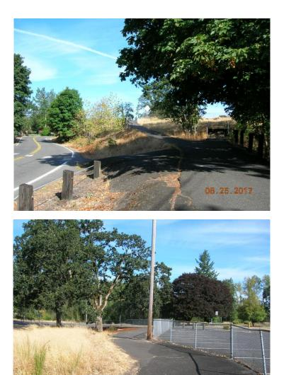
Same location as the previous photo but facing north. Note the slope along the side of the street. This is a rock outcrop that would need to be excavated to install sidewalks.
