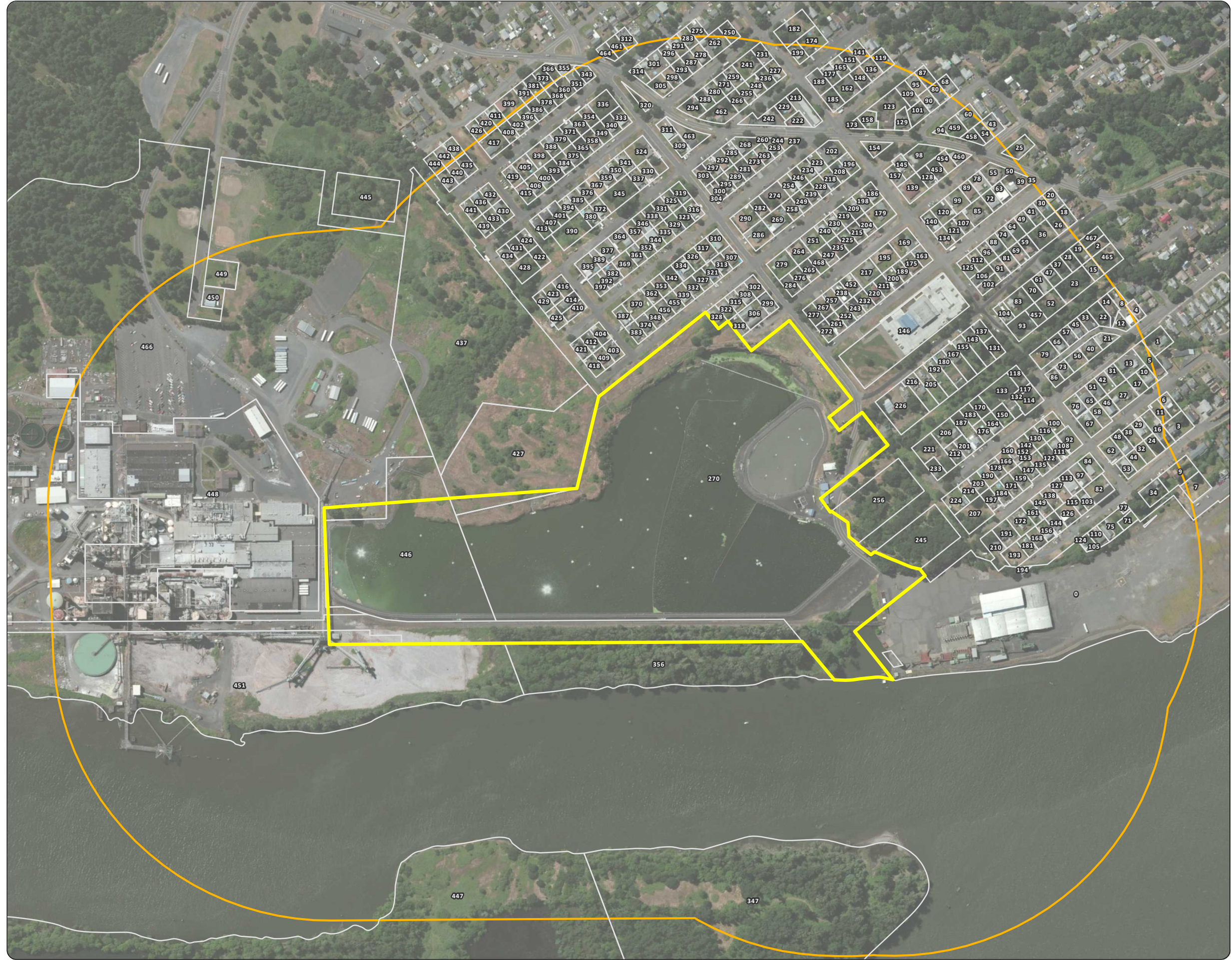
Figure 2-2 Adjacent Landowners City of St. Helens Wastewater Treatment Lagoon St. Helens, Oregon
