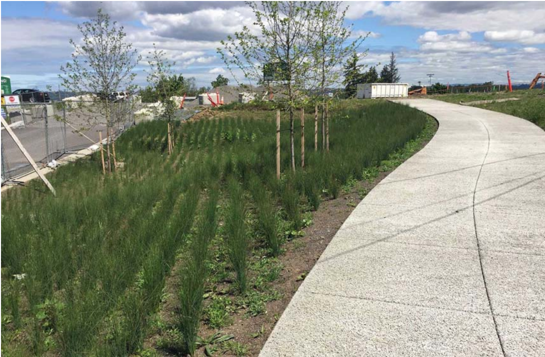
Figure 10. Completed “greenstreet” along NE 72nd Avenue.
