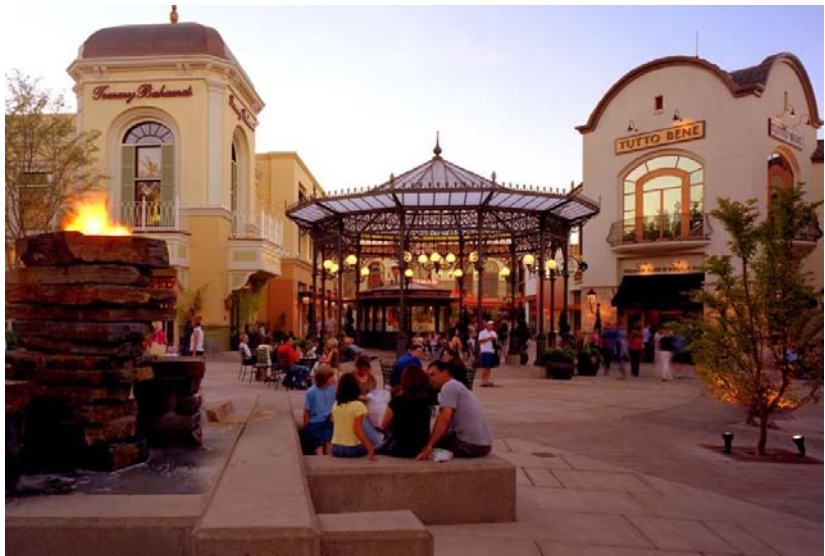
Figure 11. Bridgeport Village Development after construction complete. (Credit: The Opus Group)
