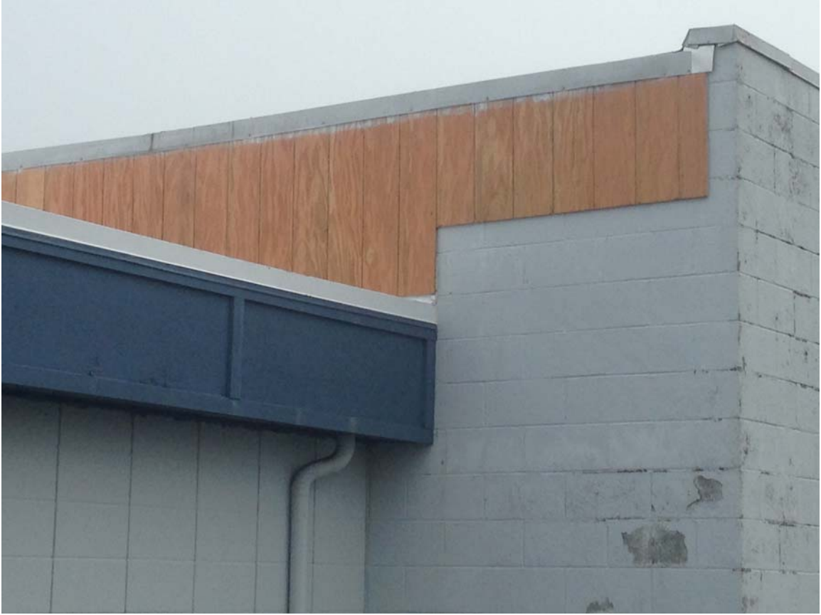
New plywood siding between garage and office.
