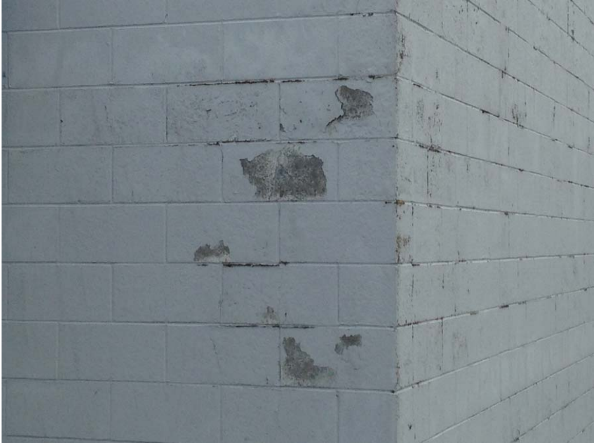
Example of peeling paint along southern exposure.
