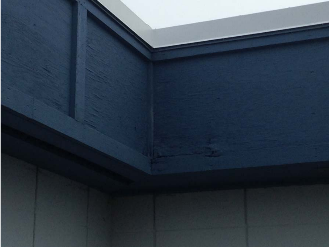
Example of dry rot along the southern exposure
