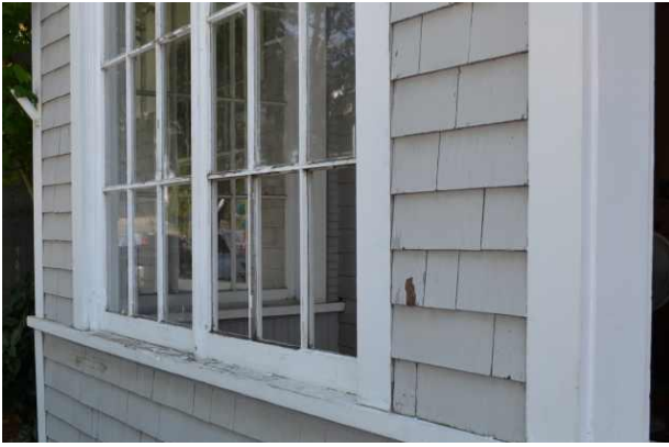
(Above) Before: Missing window panes, chipped shingles (Right) After: New post, window panes, shingles and paint
