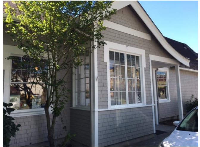
(Above) Before: Missing window panes, chipped shingles (Right) After: New post, window panes, shingles and paint
