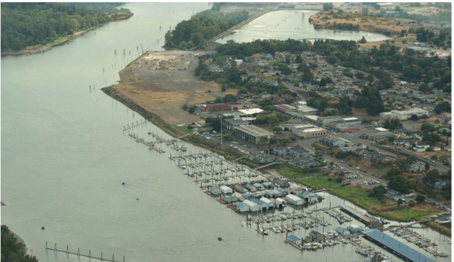
Photograph looking south from downtown St. Helens, across the Veneer Property towards the BWP Property.
