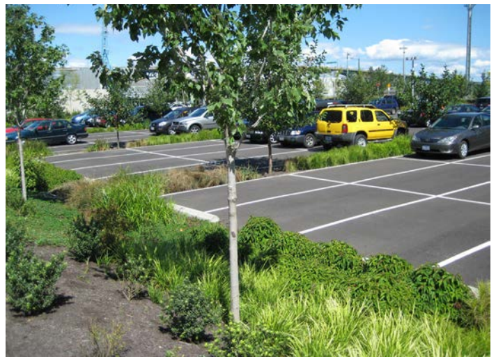
Green parking lots with trees and stormwater planters.
