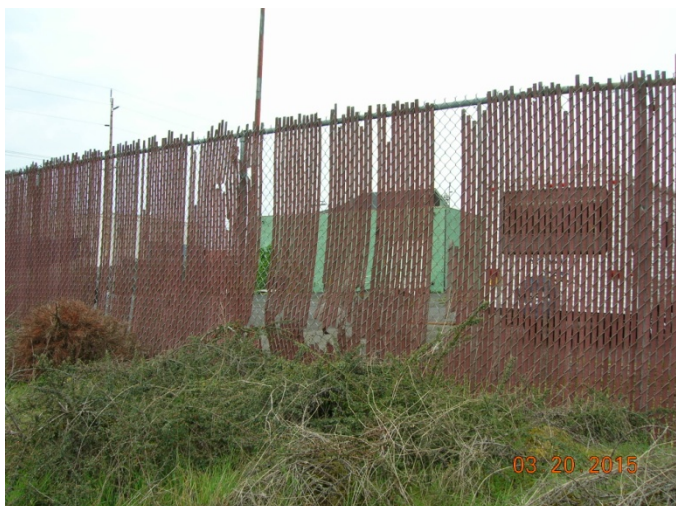
Though the existing sight-obscuring fence is in mostly good condition overall for its age, some sight obscuring measures along Cowlitz Street have seen better days.
