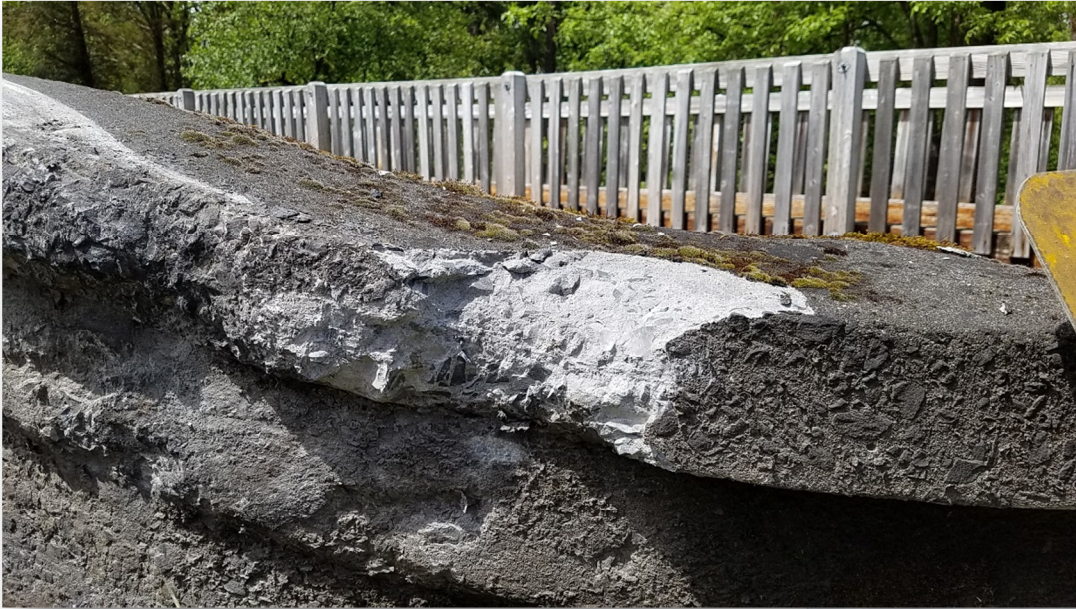
Railing Damage, Northerly End of West Railing
