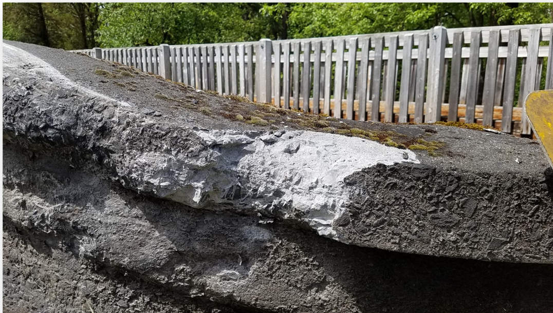
Railing Damage, Northerly End of West Railing
