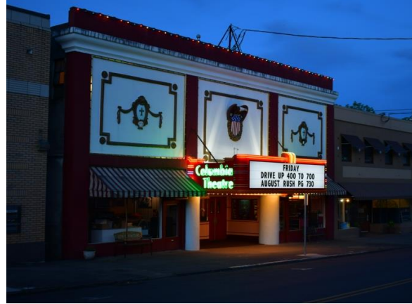
Historic Columbia Theater, renovated in 2012
