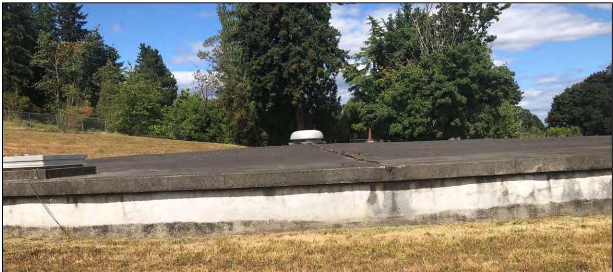
FIGURE 3-9: 2.5 MG STORAGE RESERVOIR
