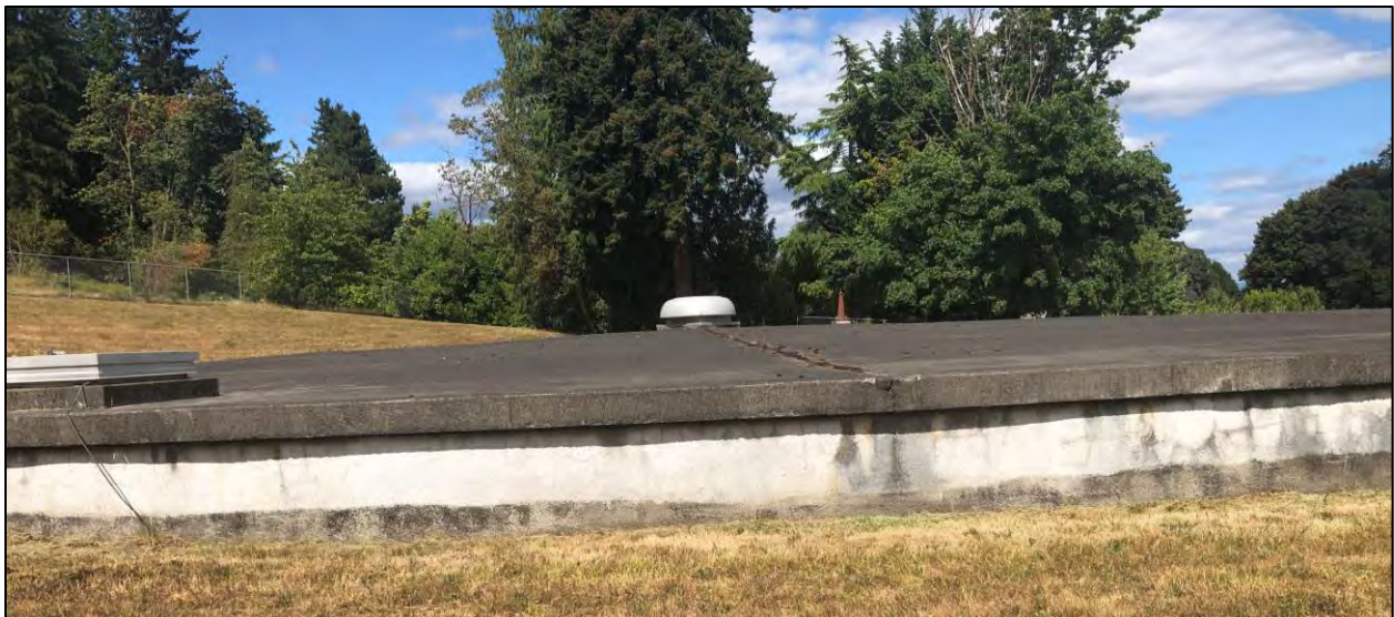
FIGURE 3-9: 2.5 MG STORAGE RESERVOIR
