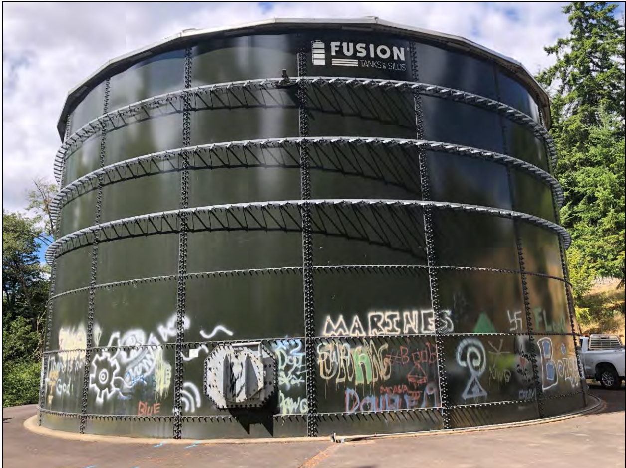
FIGURE 3-11: ELK RIDGE STORAGE RESERVOIR
