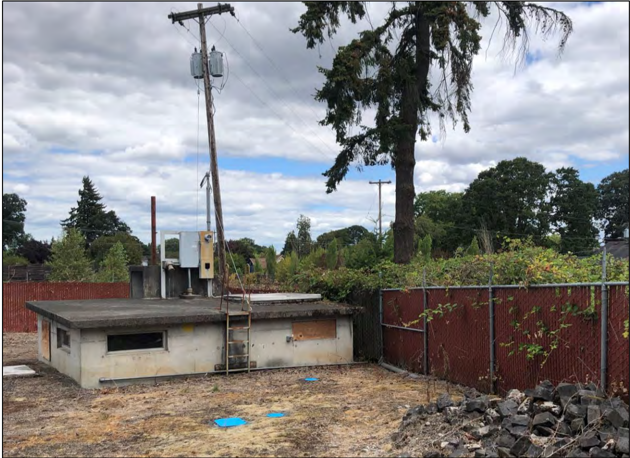
FIGURE 3-6: LEMONT BOOSTER STATION
