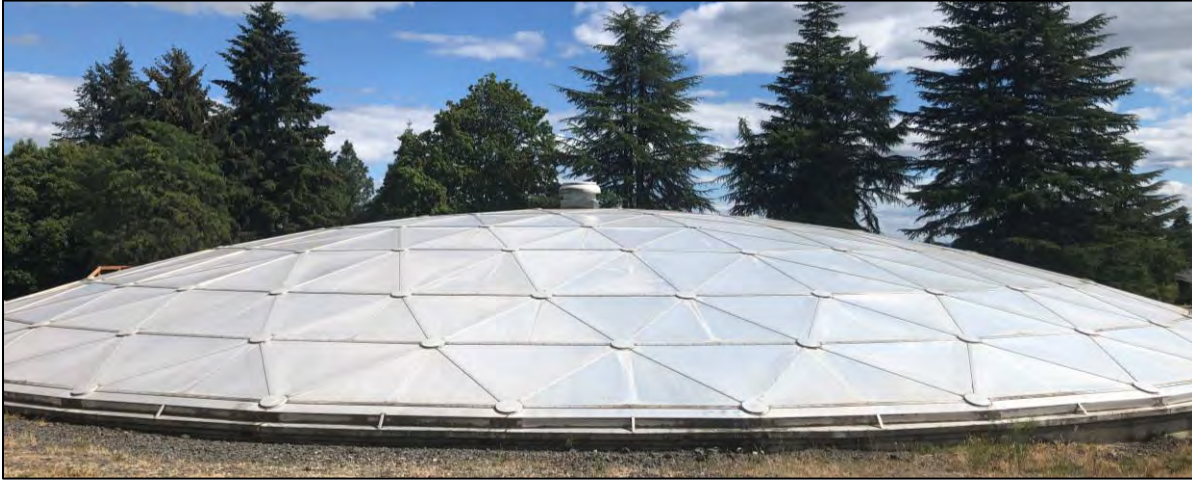
FIGURE 3-8: 2.0 MG STORAGE RESERVOIR
