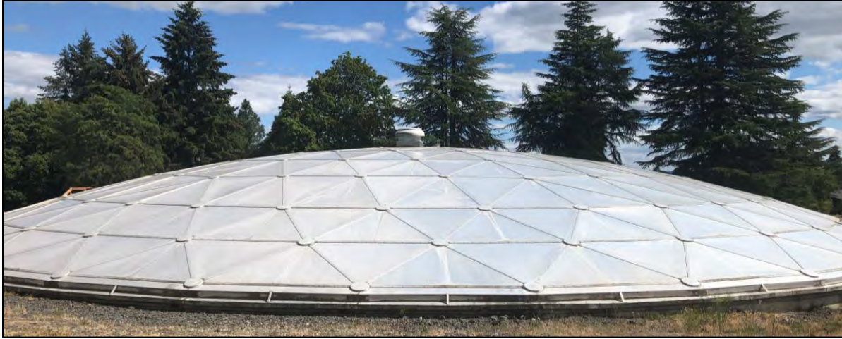
FIGURE 3-8: 2.0 MG STORAGE RESERVOIR
