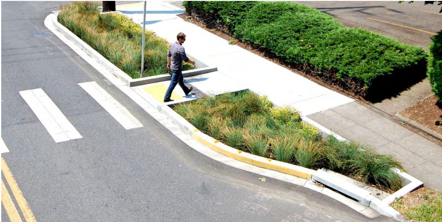
Bulb-out with stormwater facility and crosswalk
