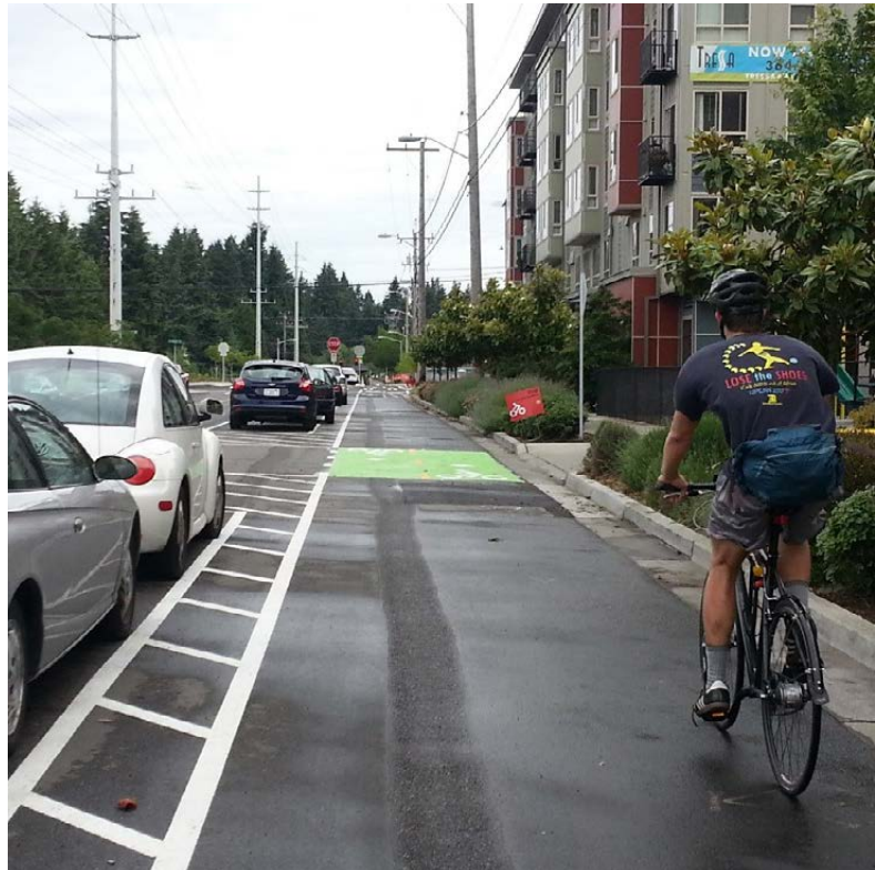
Two-way cycletrack with driveway in Seattle, WA
