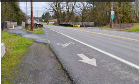
Bike path and bridge over Milton Creek
