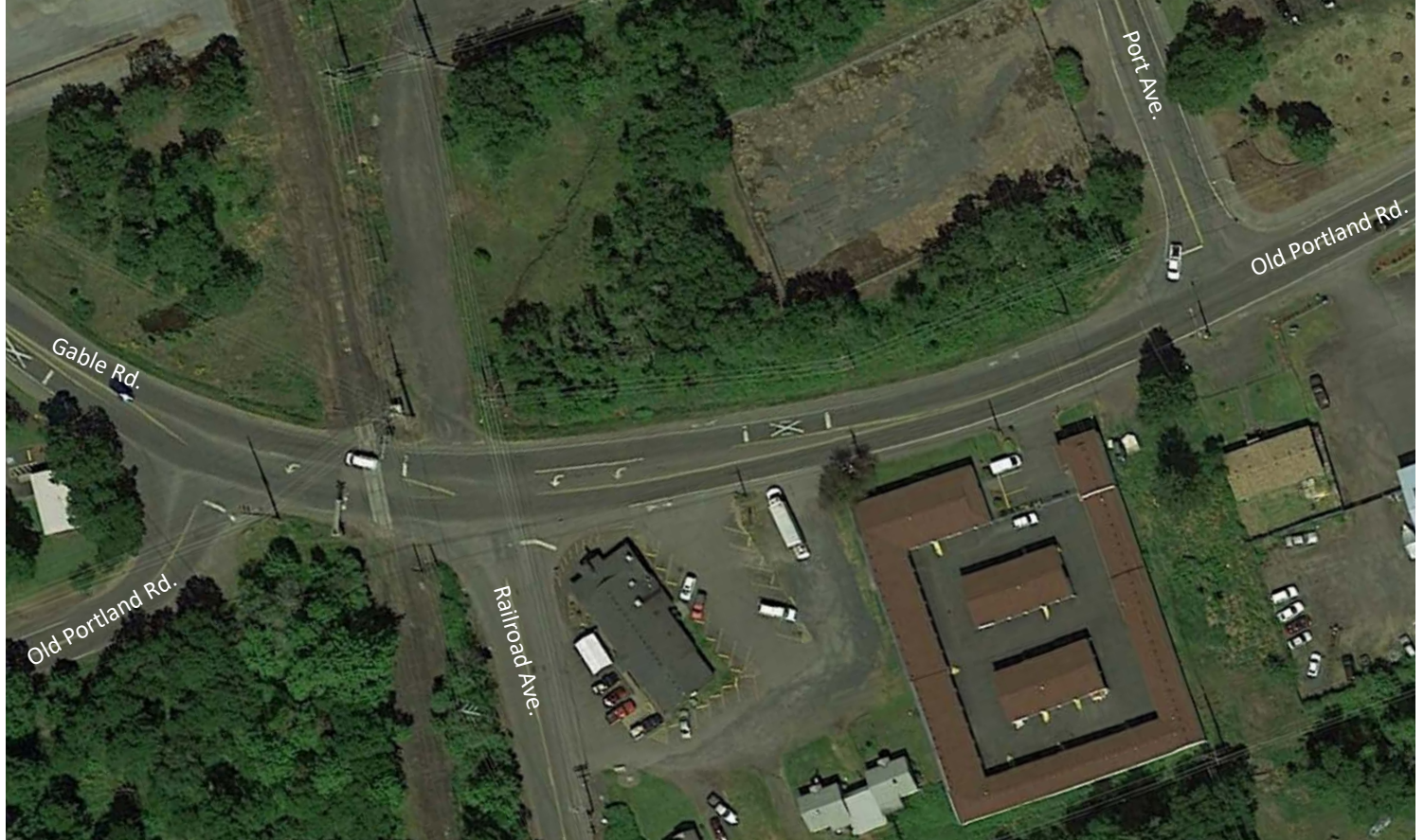
Existing conditions (image: Google Earth)
