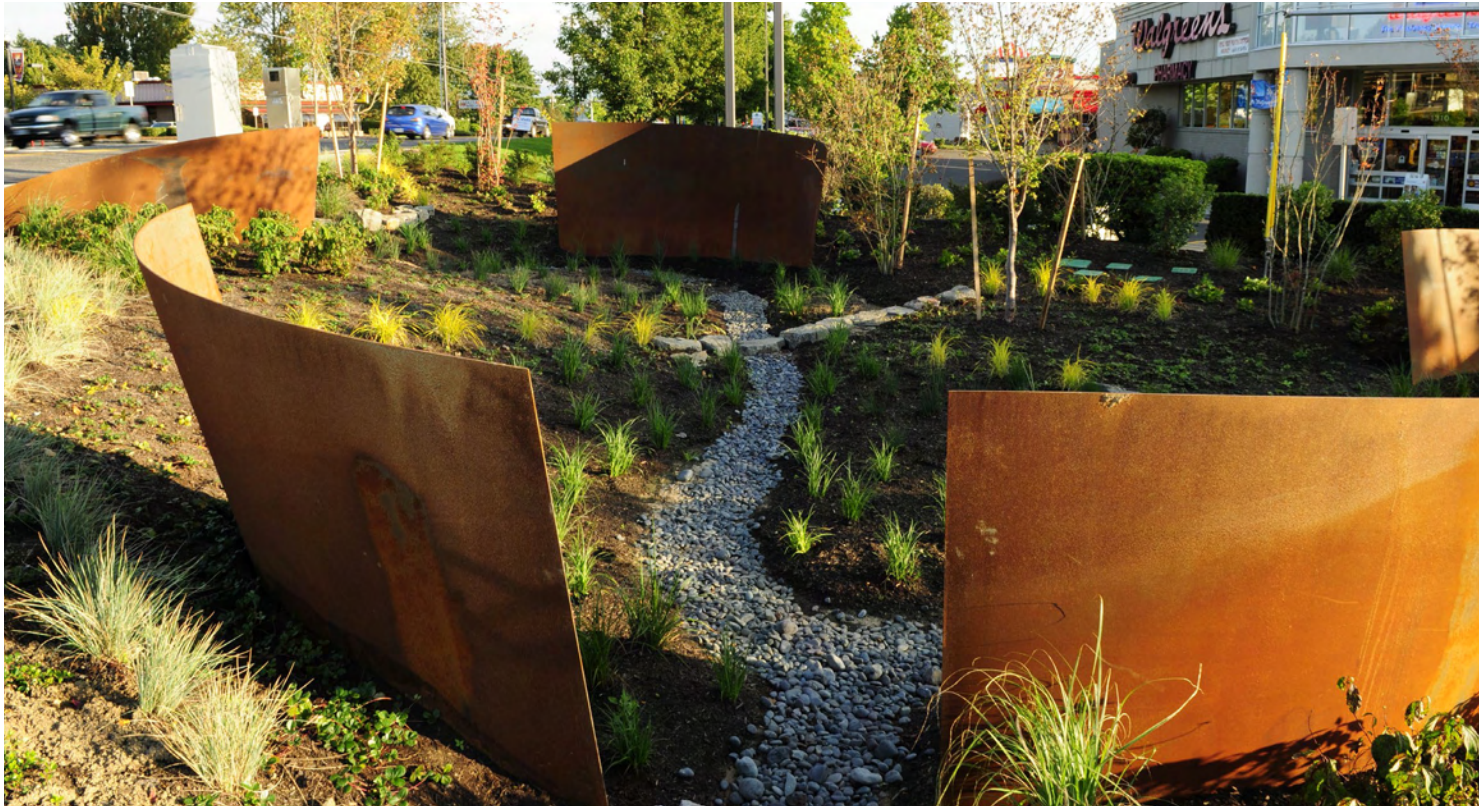
The Warner Milne Rain Garden in Oregon City collects stormwater and runoff from adjacent surfaces
