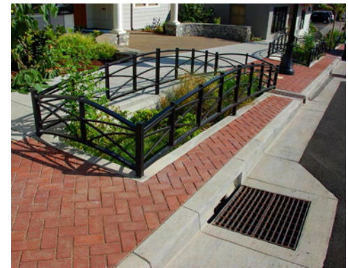
Brick and concrete paving
