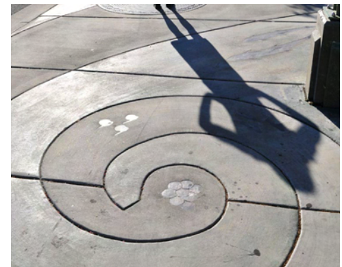
Decorative concrete paving
