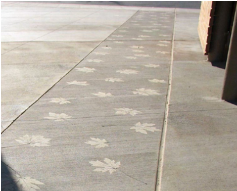
Stamped concrete paving
