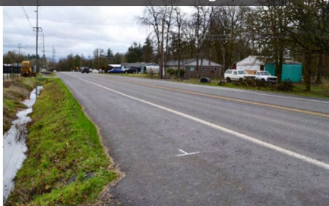
Grass conveyance ditch and bike lane on Gable Road looking north
