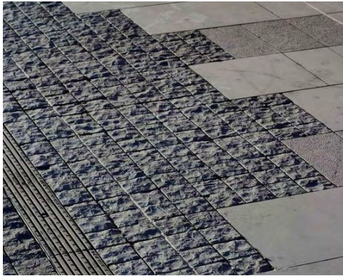
Concrete unit pavers and cobblestones
