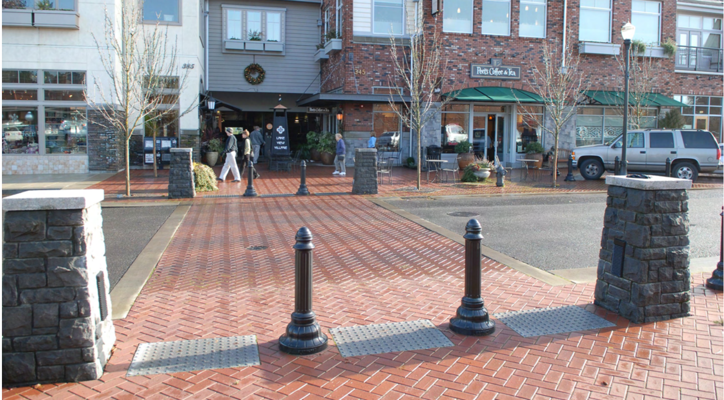
Bollards, stone markers and the use of brick makes a mid-block crossing in Lake Oswego, OR more noticeable
