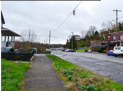
South 1st Street looking south
