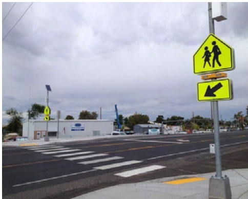
Crossing with Rectangular Rapid Flashing Beacon
