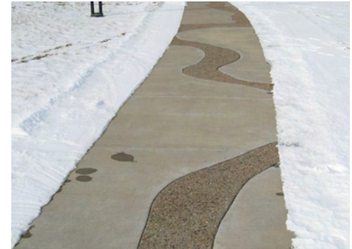
Concrete and aggregate paving
