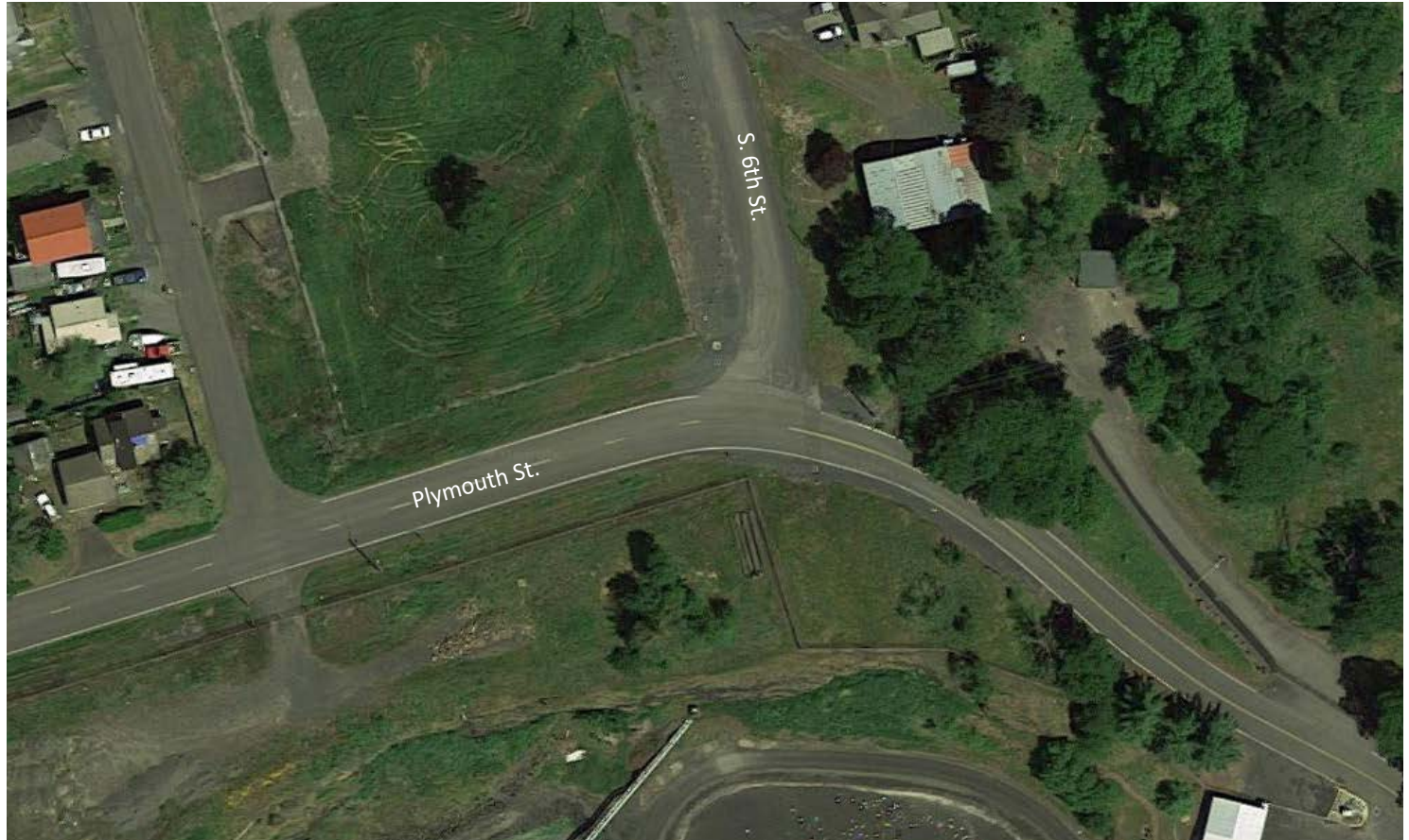
Existing conditions (image: Google Earth)
