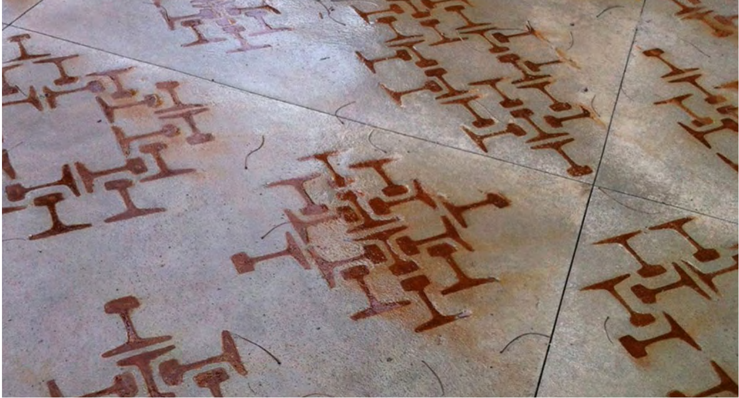
Stenciled concrete paving
