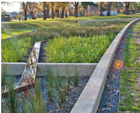
Artful rainwater conveyance in Melbourne, Australia
