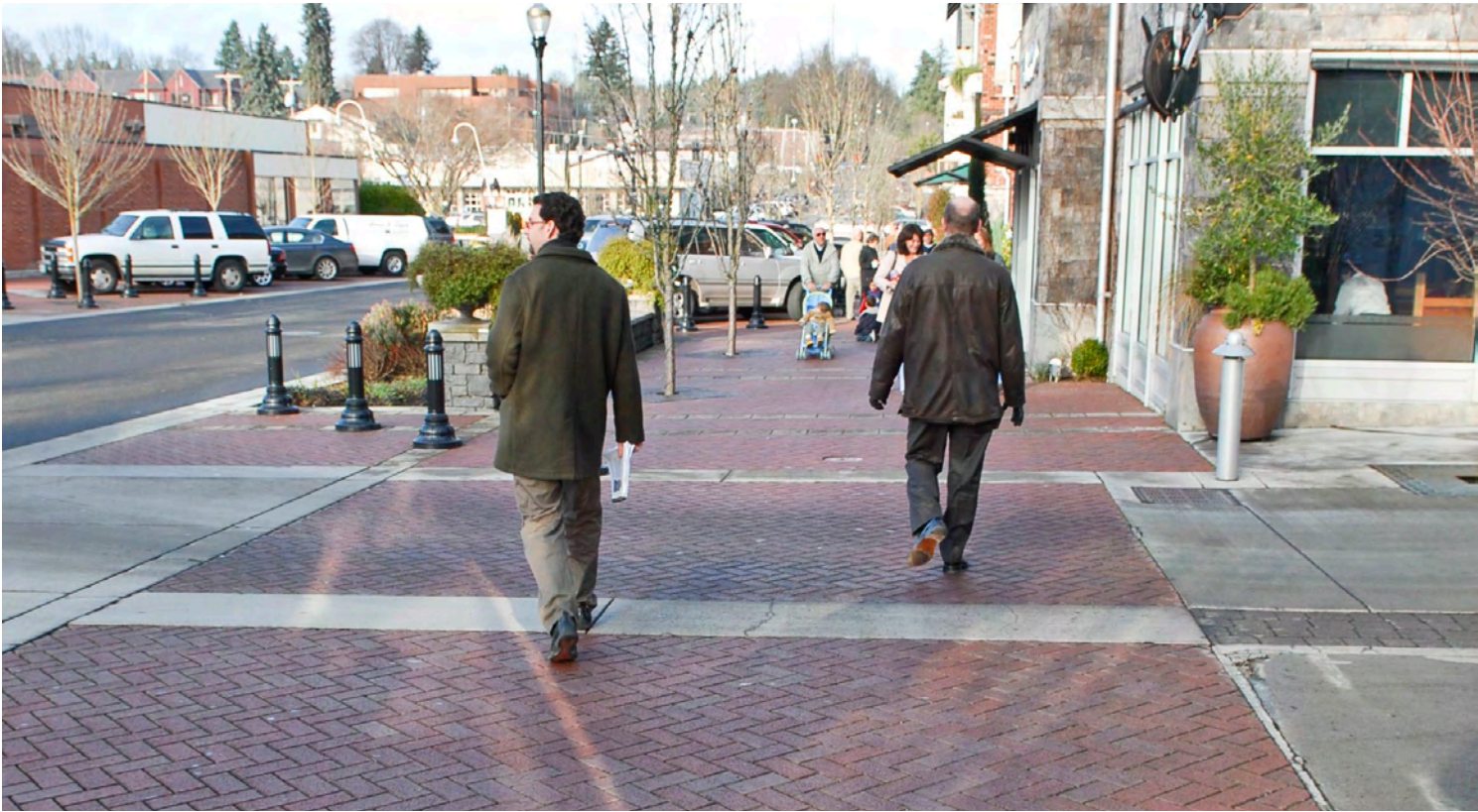
Brick and paving bands suggest a change of conditions
