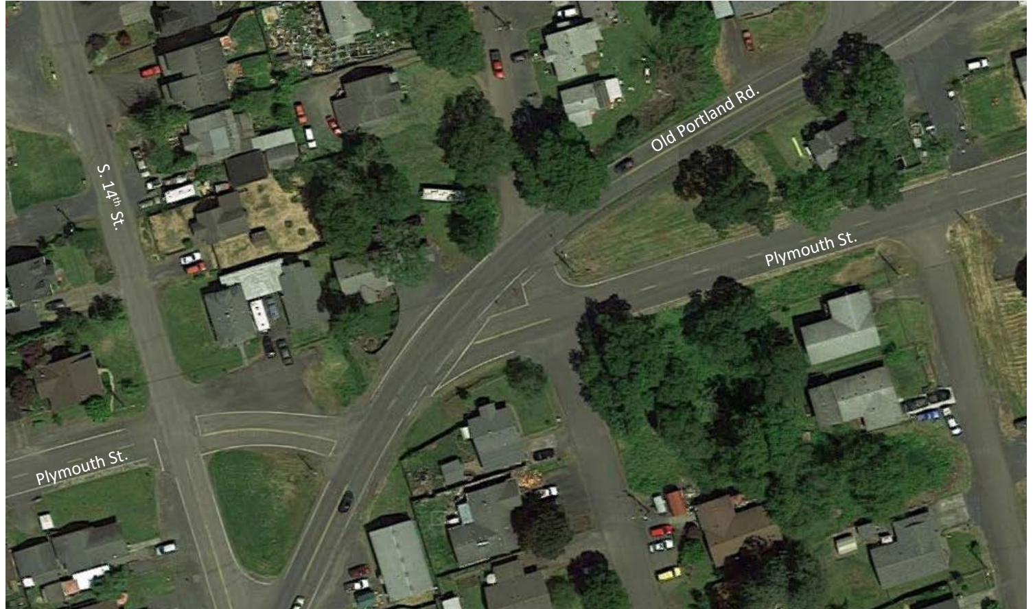
Existing conditions (image: Google Earth)
