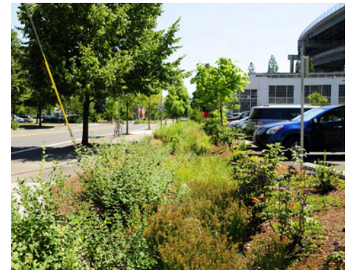
Mature stormwater planter along Water Avenue
