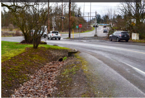
Conveyance ditch on Old Portland Road
