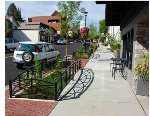
Stormwater planter with railing in Lake Oswego, OR
