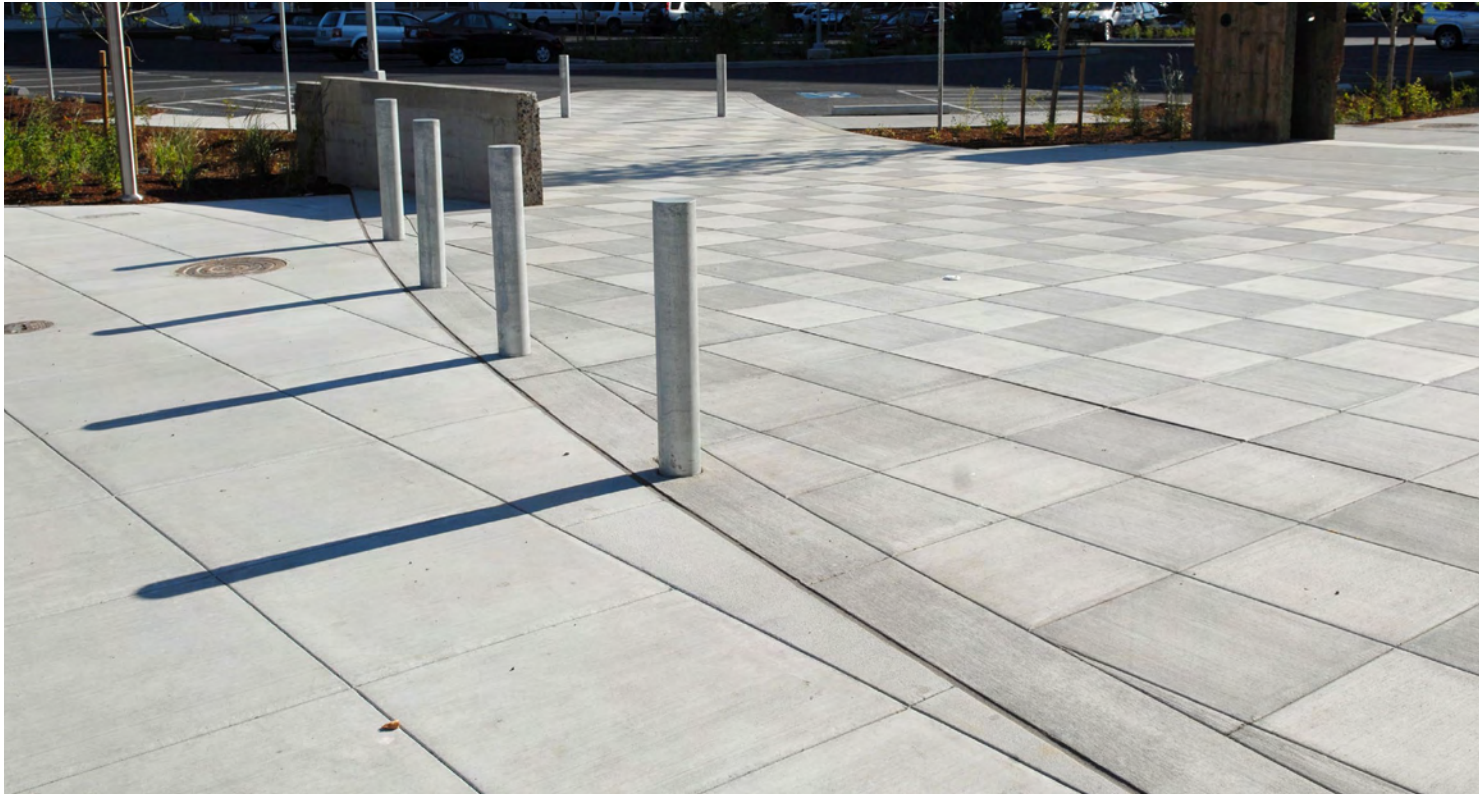
Scored concrete paving
