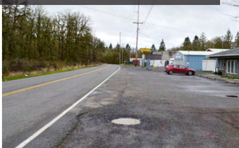
Gravel shoulder on Old Portland Road
