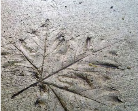
Stamped concrete paving
