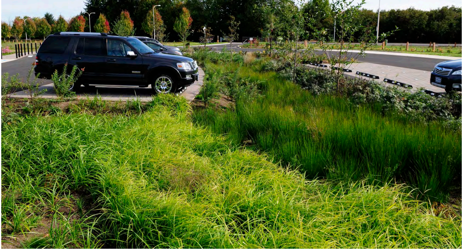
Permeable paving parking stalls at Graham Oaks Nature Park in Wilsonville, OR
