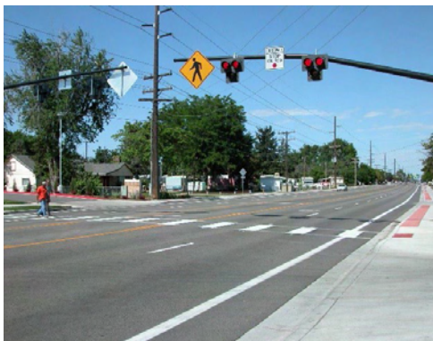
Crossing with Pedestrian Hybrid Beacon
