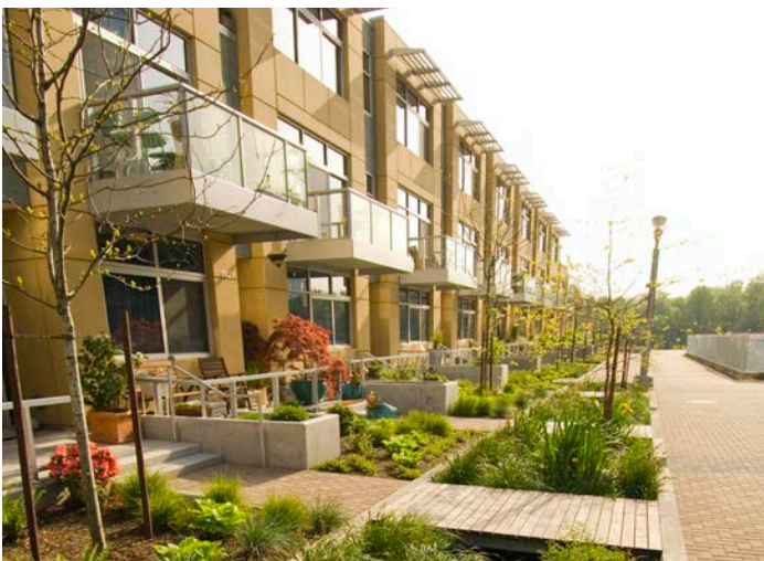
Low-impact stormwater treatment along pedestrian accessway.
