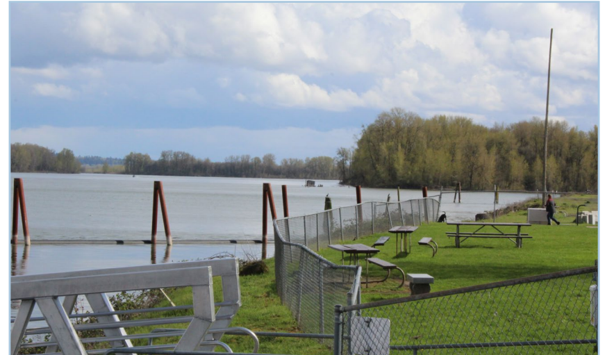
4 Community members feel like the river's edge is uninviting. They dislike the chain link fence and the uncomfortable walking environment.
