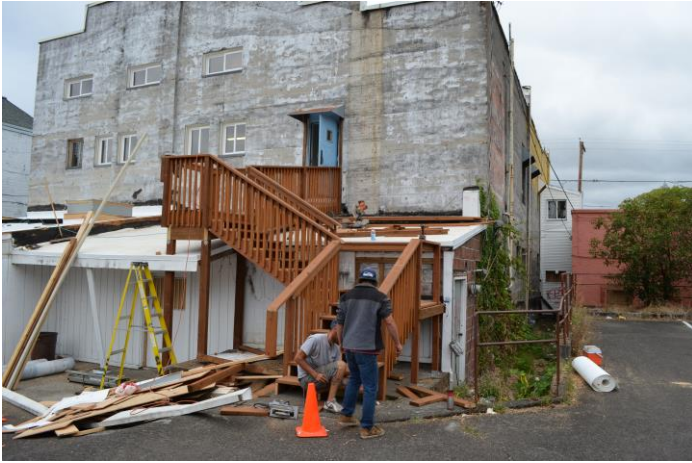
During & After: Old staircase removed and being rebuilt. New roofing on secondary building and 8 new white vinyl windows. Stained glass replaced on front of building.
