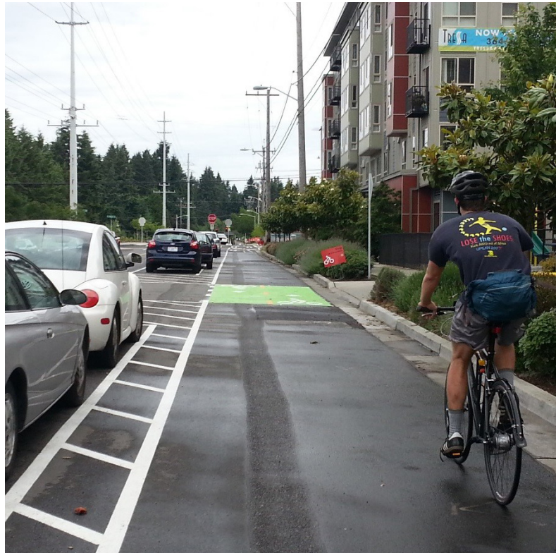
Two-way cycletrack with driveway in Seattle, WA
