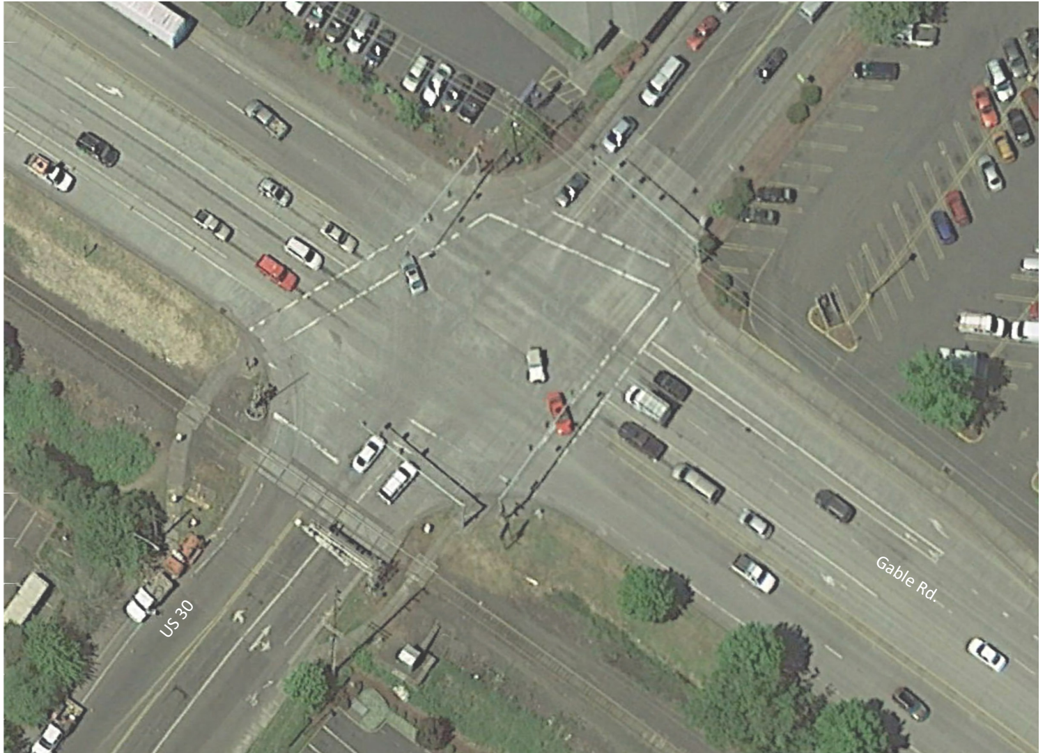
Existing conditions (image: Google Earth)
