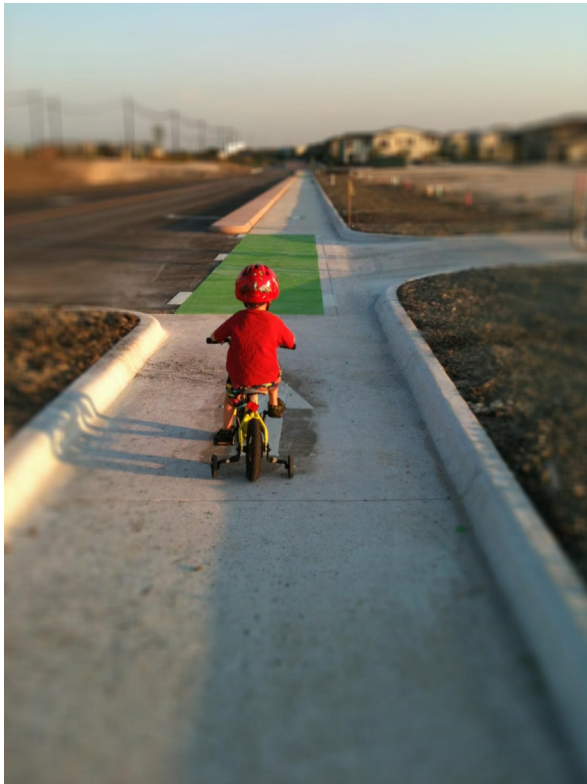
Grade-separated cycletrack with driveway in Austin, TX
