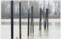
MATERIAL. WEATHERED WOOD
