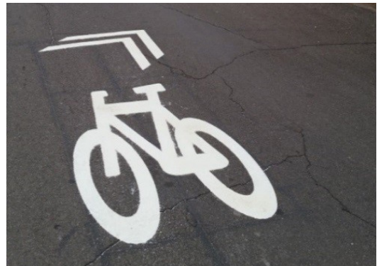
Directional shared lane marking (not FHWA approved)
