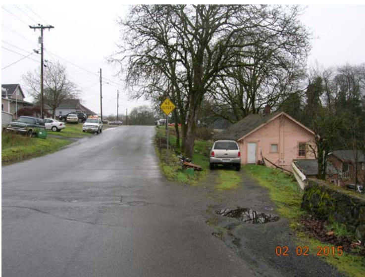
Photo taken from the S. 4 th Street R.O.W. looking south. This is also the S. 4 th Street/Tualatin Street intersection.
