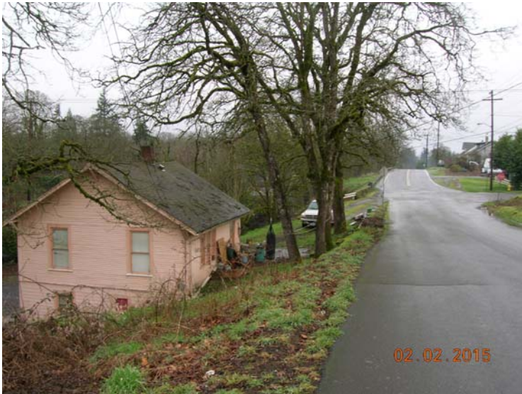
Photo taken from the S. 4 th Street R.O.W. looking north.
