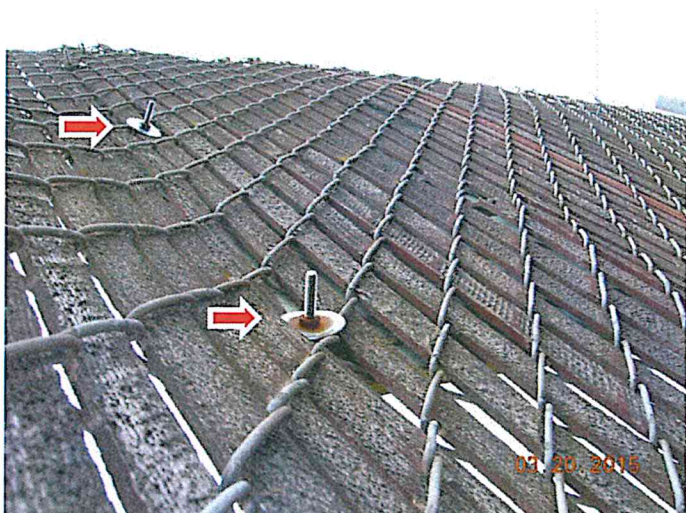
This picture shows the method of attachment of the wood signs noted in the staff report.
