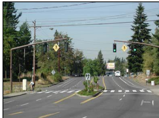
Signalized crossing for a roadway with ADT over 15,000
