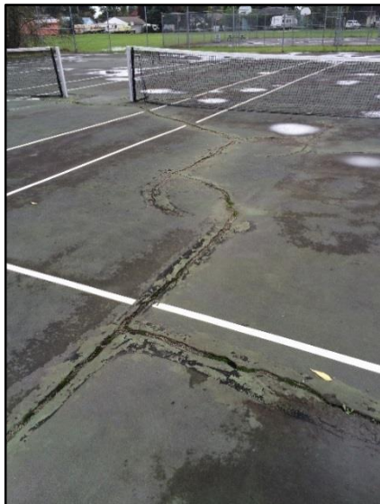
Tennis court cracks and previous attempts to repair cracks
